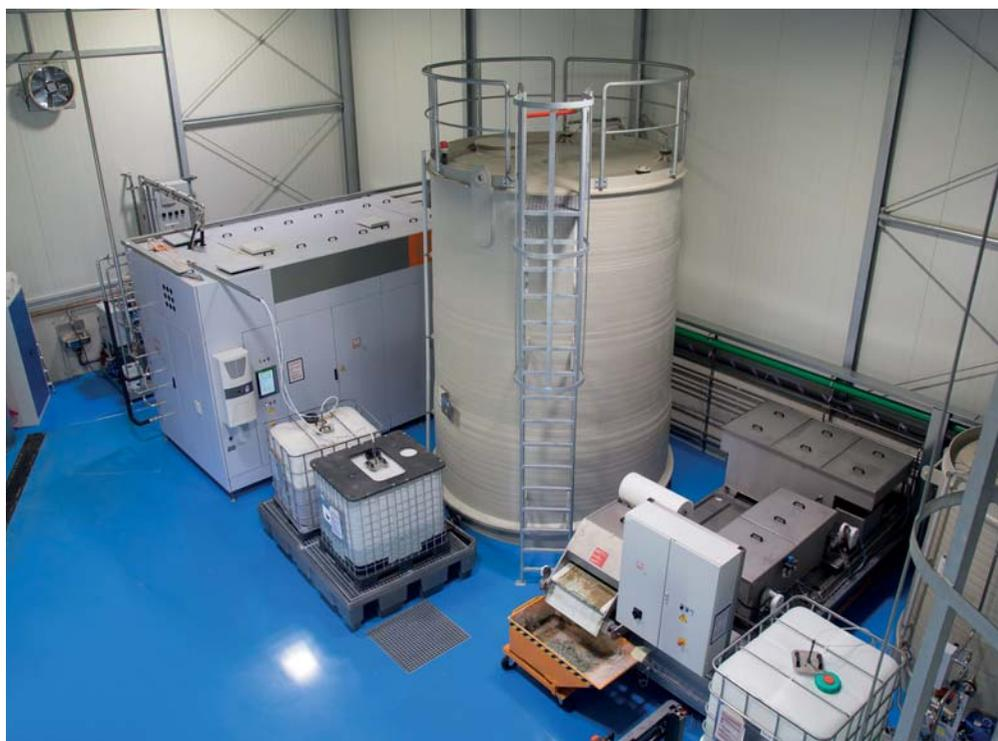
current or counter-current resin-based lines for the treatment of demineralised water, as well as special systems for acid recovery. Ultrafiltration systems, coalescence oil separators, and centrifuges for the treatment of degreasing and phosphodegreasing tanks complete the company's range. The main innovation, however, are its evaporators combining mechanical compression with
